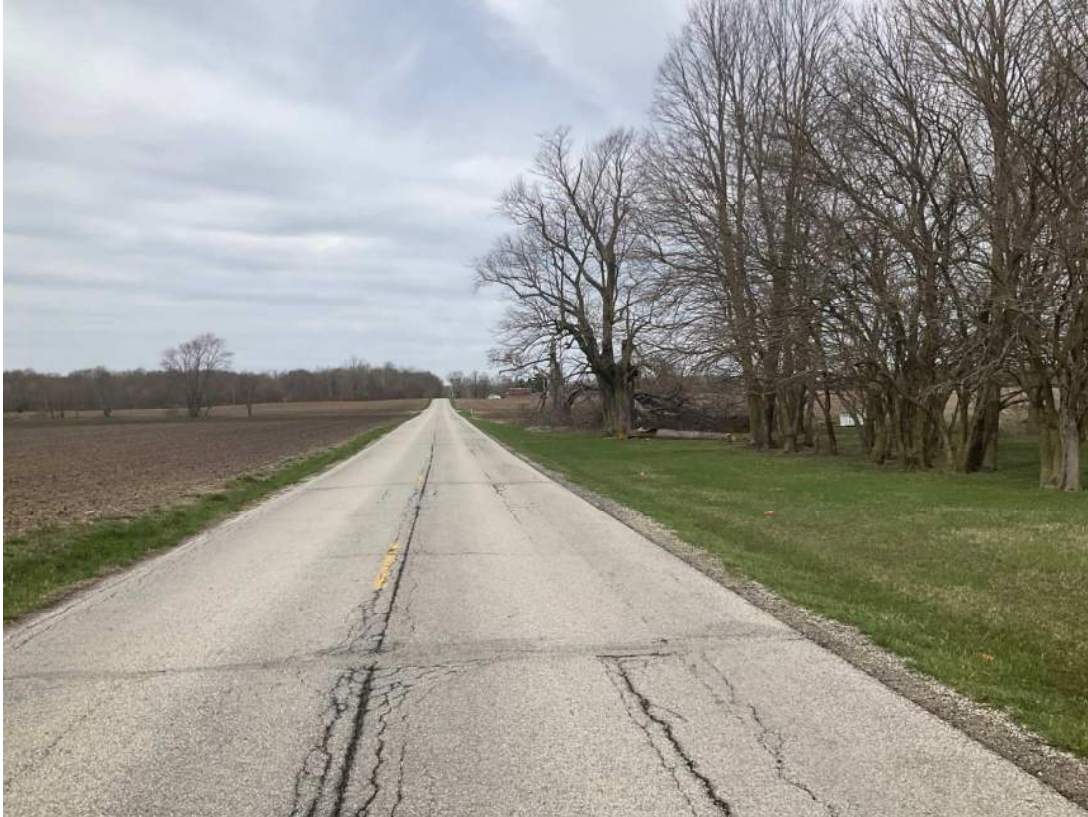
15. Looking NW from East 281 st Street at roadway.
