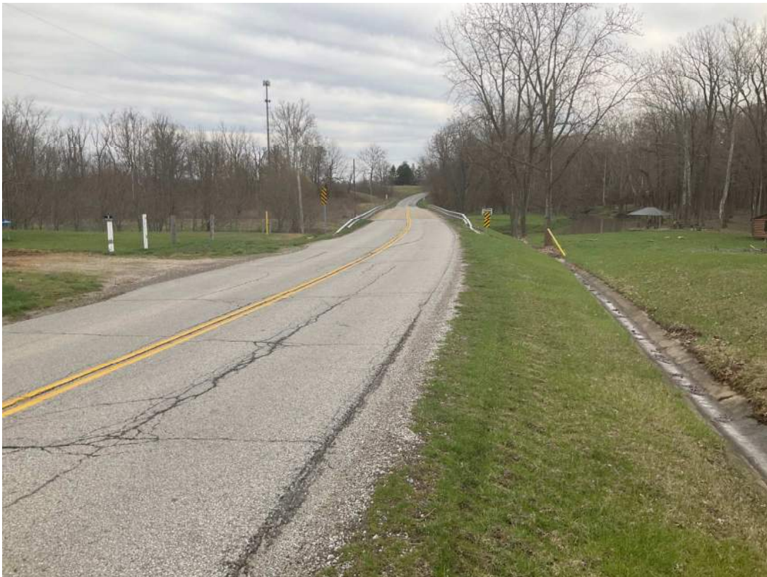
6. Looking northeast (NE) along the south side of East 281 st Street.
