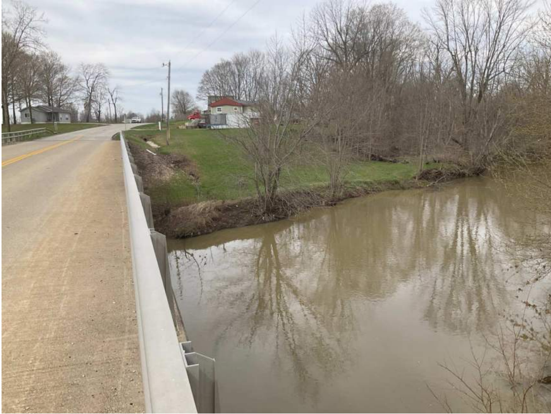
11. Looking W from the bridge that spans Cicero Creek.
