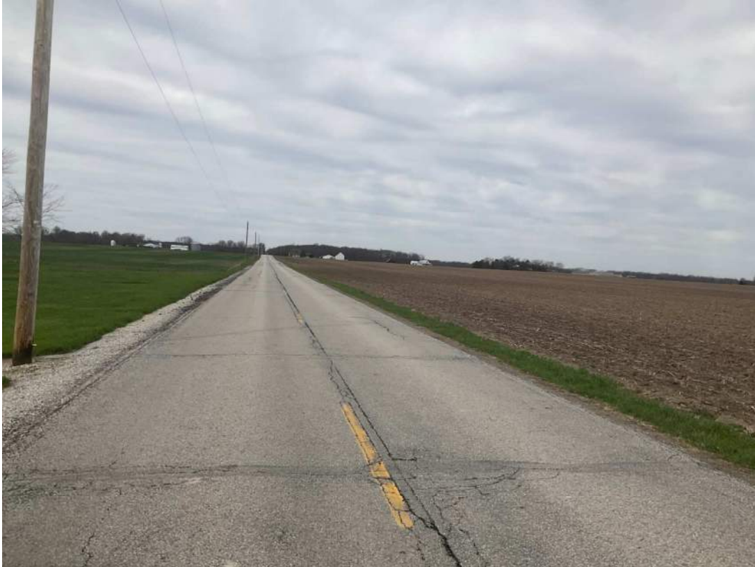
19. Looking W from East 281 st Street at roadway.
