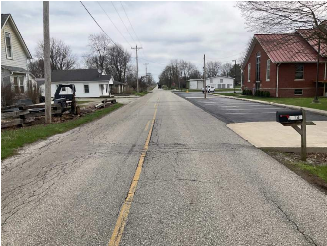
32. Looking E at the East 281 st Street / SR 213 Intersection (eastern terminus).
