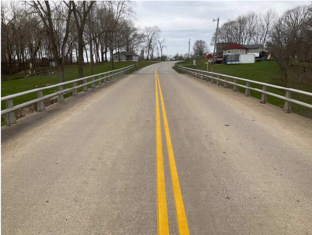
9. Looking southwest (SW) from the bridge that spans Cicero Creek.
