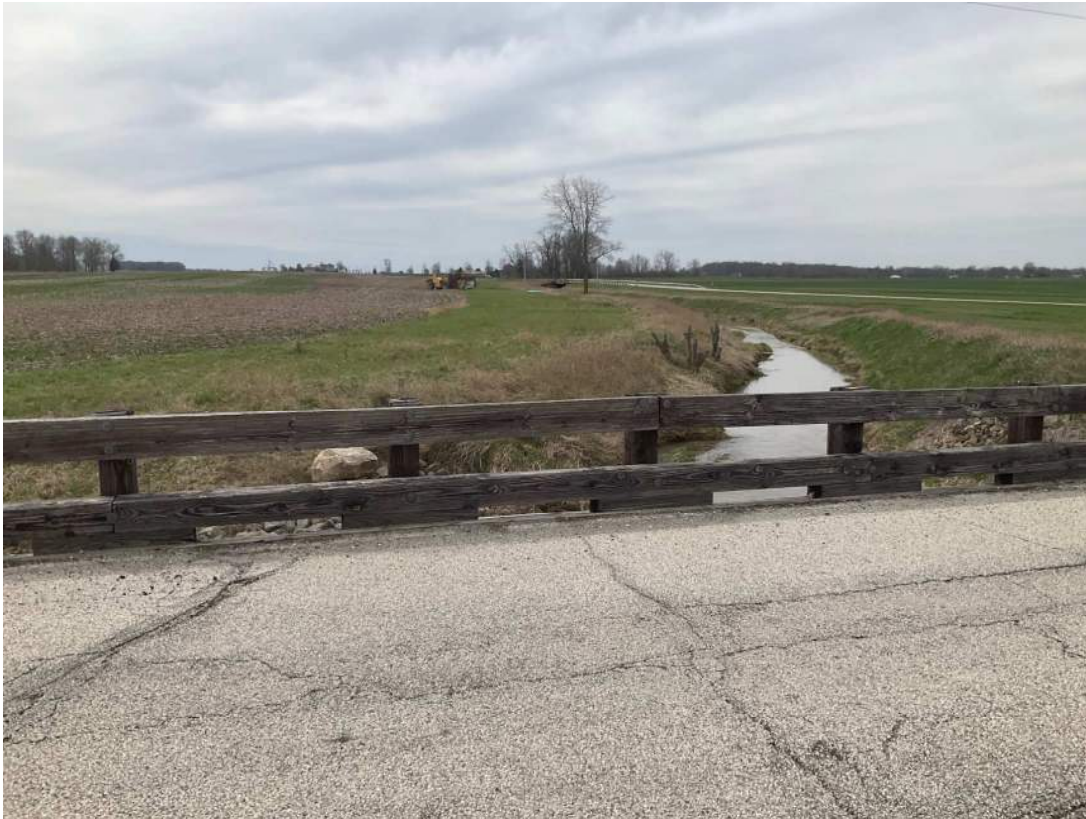
27. Looking SW from bridge that spans Weasel Creek.
