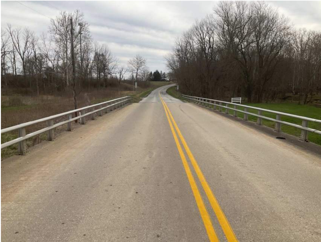
7. Looking E along the bridge that spans Cicero Creek.
