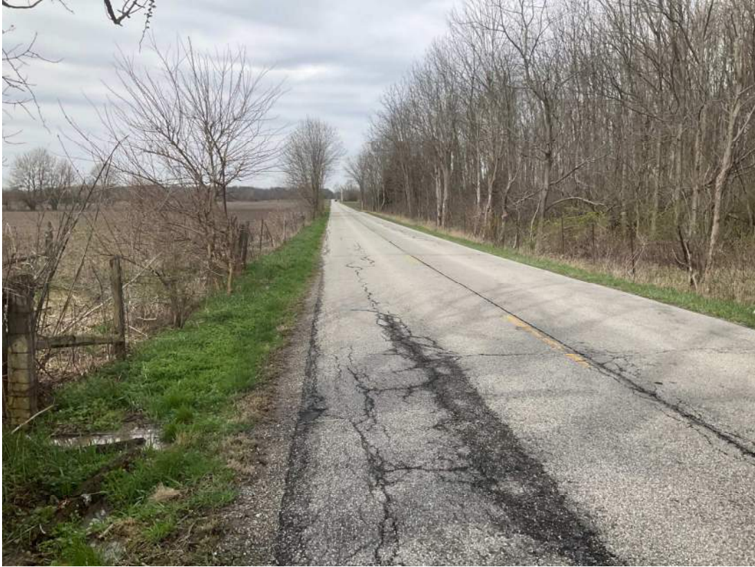
17. Looking W from East 281 st Street at roadway.
