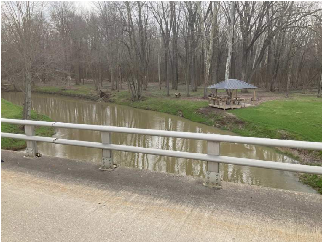
8. Looking southeast (SE) from the bridge that spans Cicero Creek.
