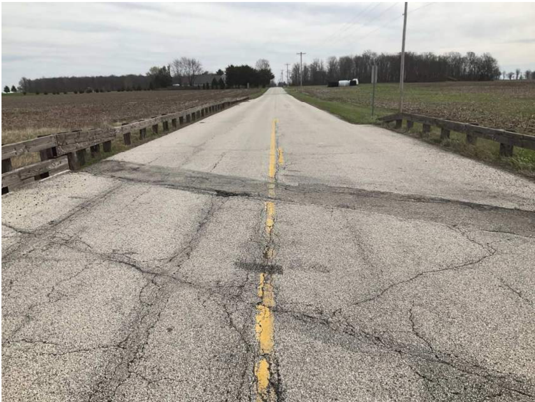
26. Looking E from the bridge that spans Weasel Creek.
