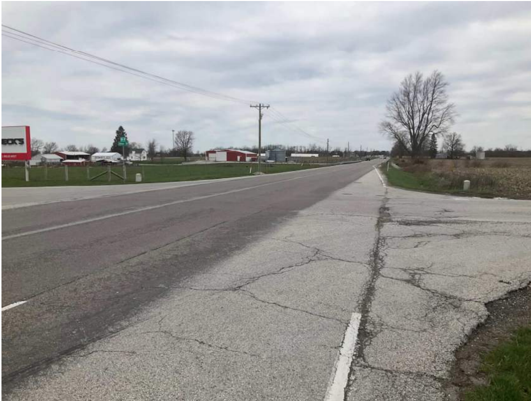
1. Looking northwest (NW) at the East 281 st Street / SR 19 Intersection (western terminus).
