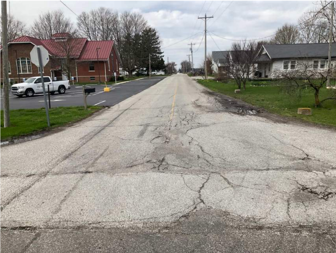
35. Looking W at the eastern terminus.
