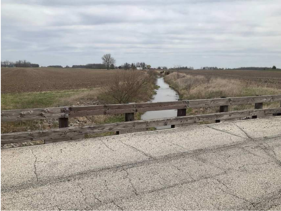
25. Looking NE from the bridge that spans Weasel Creek.
