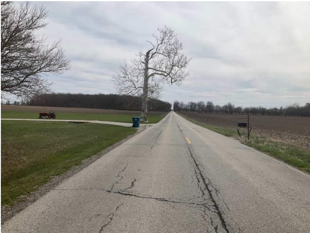
16. Looking E from East 281 st Street at roadway.
