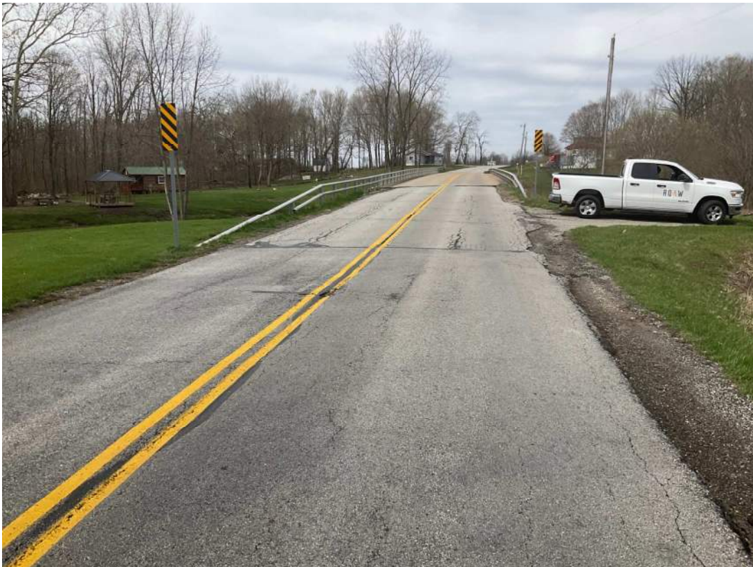
12. Looking SW towards the bridge that spans Cicero Creek.
