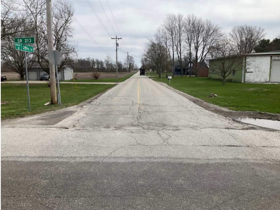
33. Looking E away from the eastern terminus.
