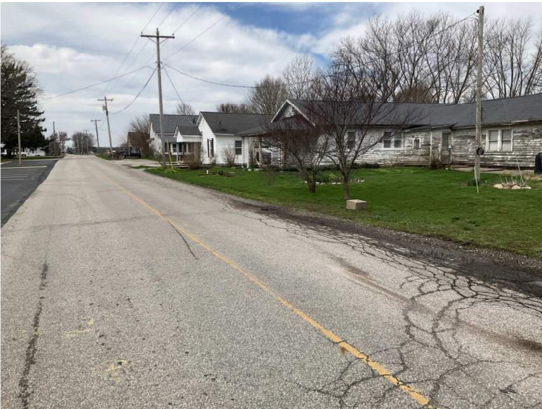
36. Looking NW from East 281 st Street at roadway (eastern terminus).
