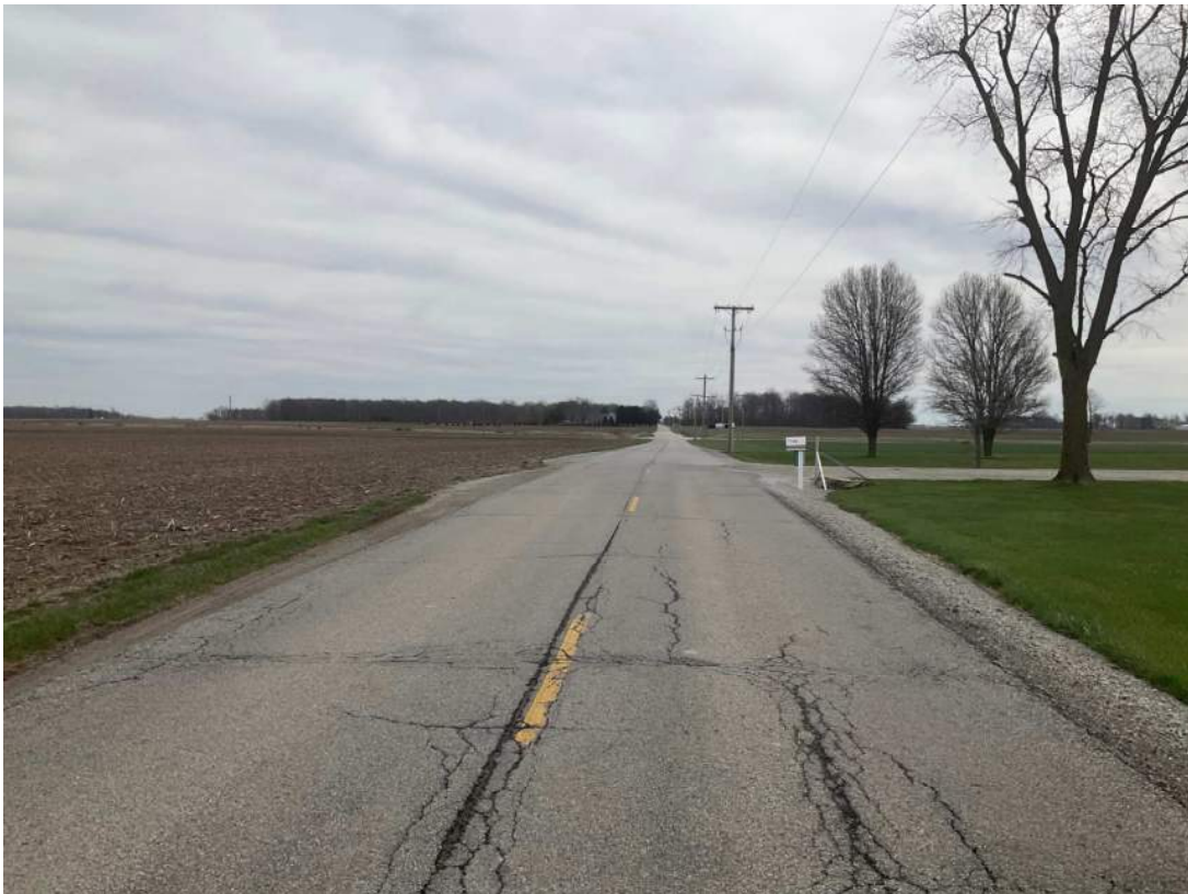
20. Looking E from East 281 st Street at roadway.
