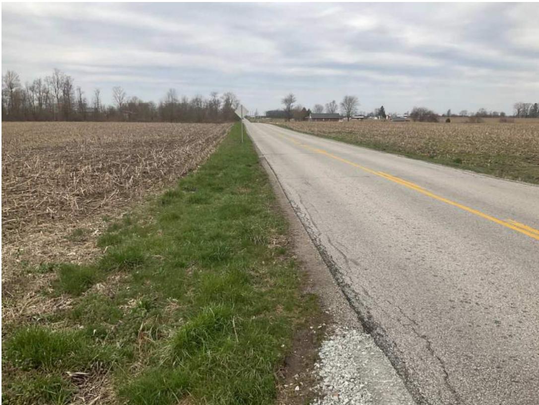
4. Looking south (S) from the East 281 st Street / Ott Road Intersection.
