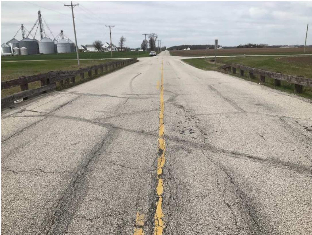
28. Looking W from bridge that spans Weasel Creek.
