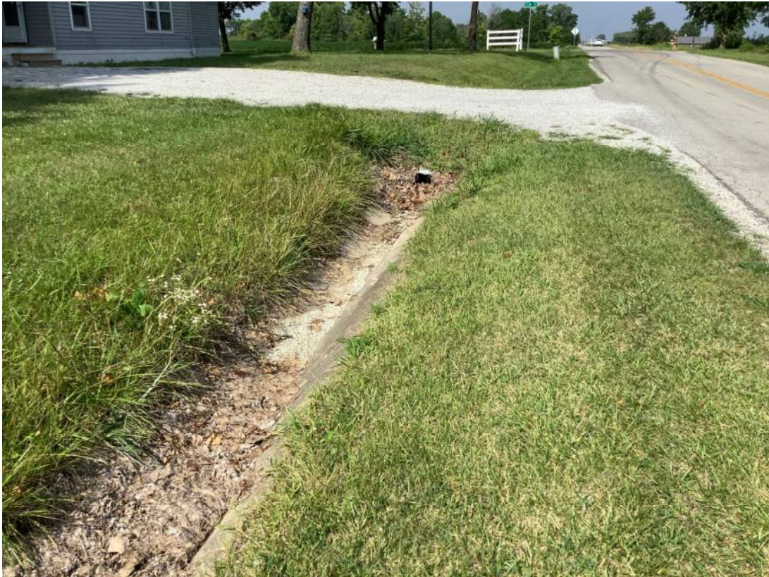
33. Facing southwest just south of 281 st St. looking at RSD 5 and maintained roadside. Photo taken 08/08/2023.
