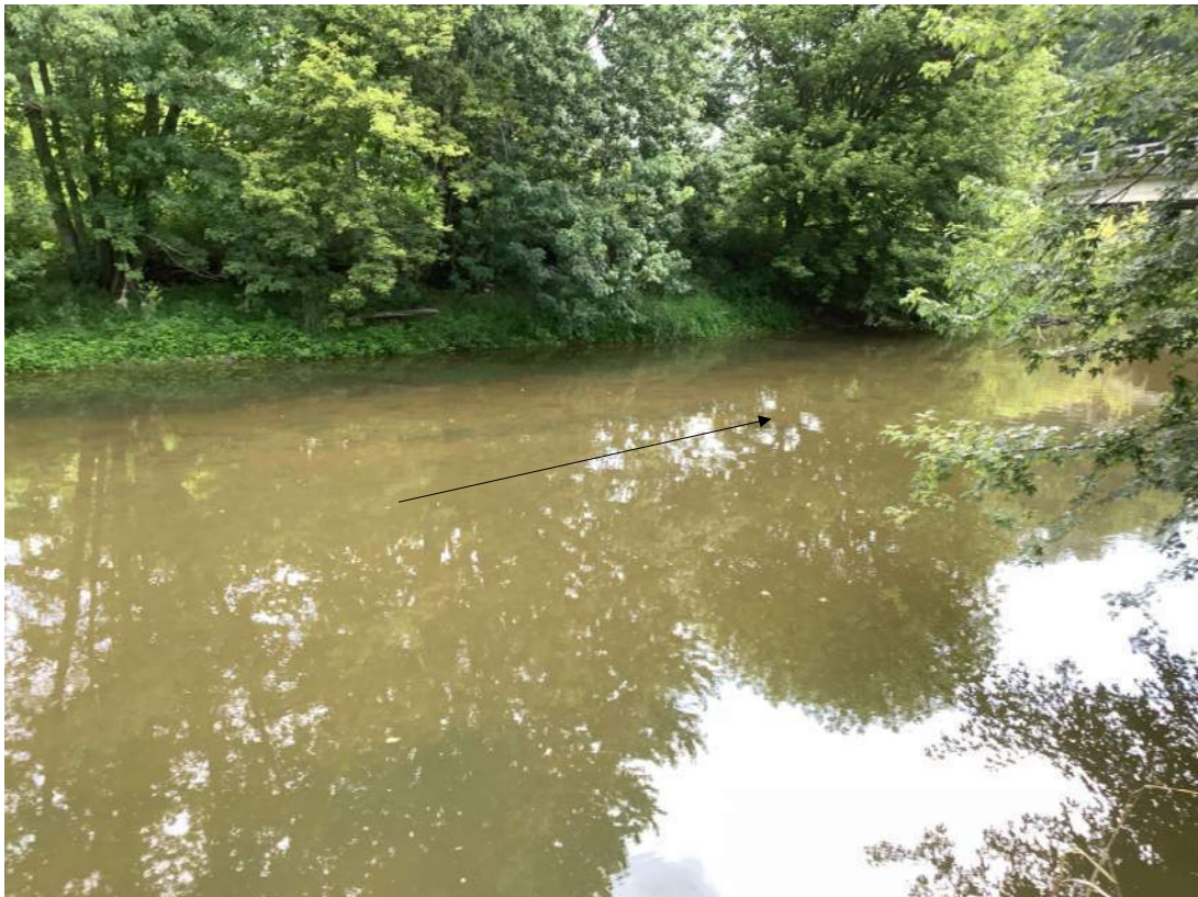
42. Facing east looking at Cicero Creek upstream of structure NBI: 400046. Photo taken 08/08/2023.
