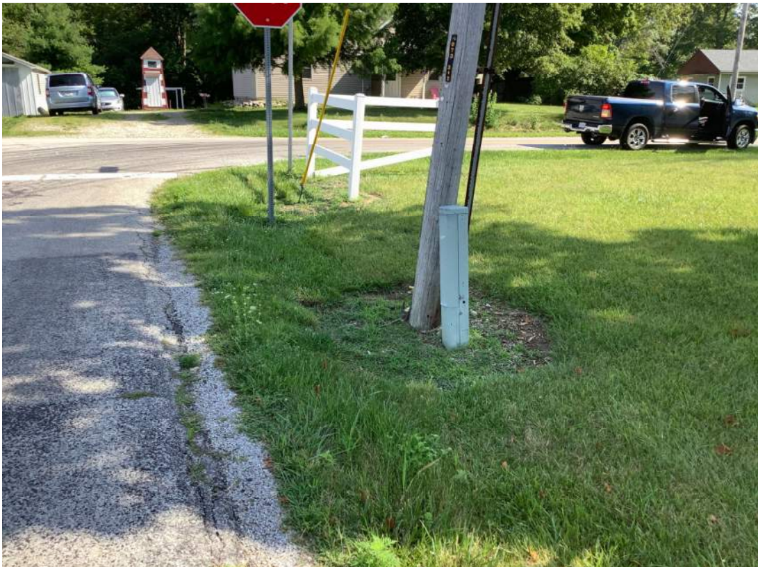
30. Facing northeast just south of 281 st St. looking at maintained roadside. Photo taken 08/08/2023.
