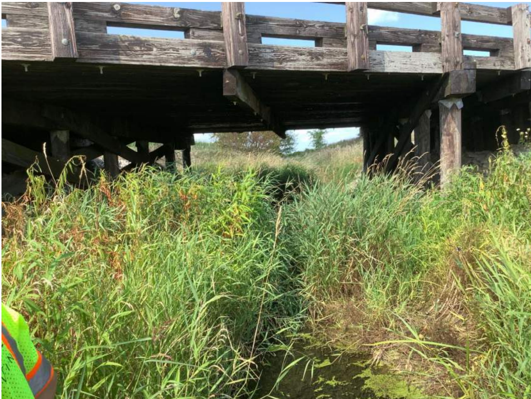
134. Facing northeast just south of 281 st St. looking at Weasel Creek and Structure 29-00066 which carries 281 st St. over Weasel Creek. Photo taken 08/08/2023.
