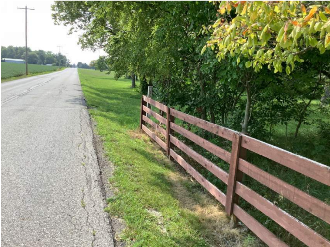
141. Facing west just north of 281 st St looking at maintained roadside and surroundings. Photo taken 08/08/2023.
