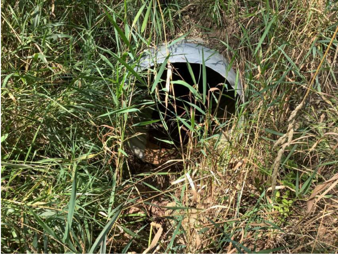
97. Facing north just south of 281 st St. looking at drainage outlet of structure. Photo taken 08/08/2023.
