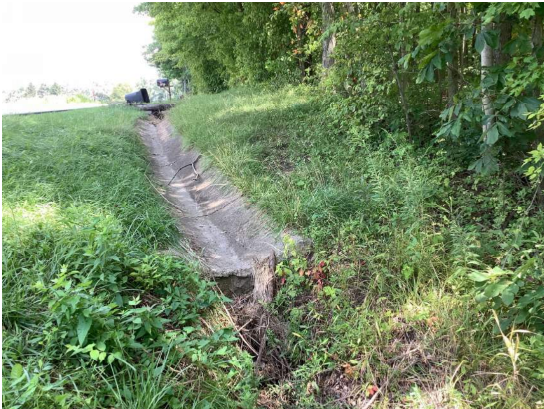
92. Facing east just south of 281 st St. looking at RDS 7. . Photo taken 08/08/2023.
