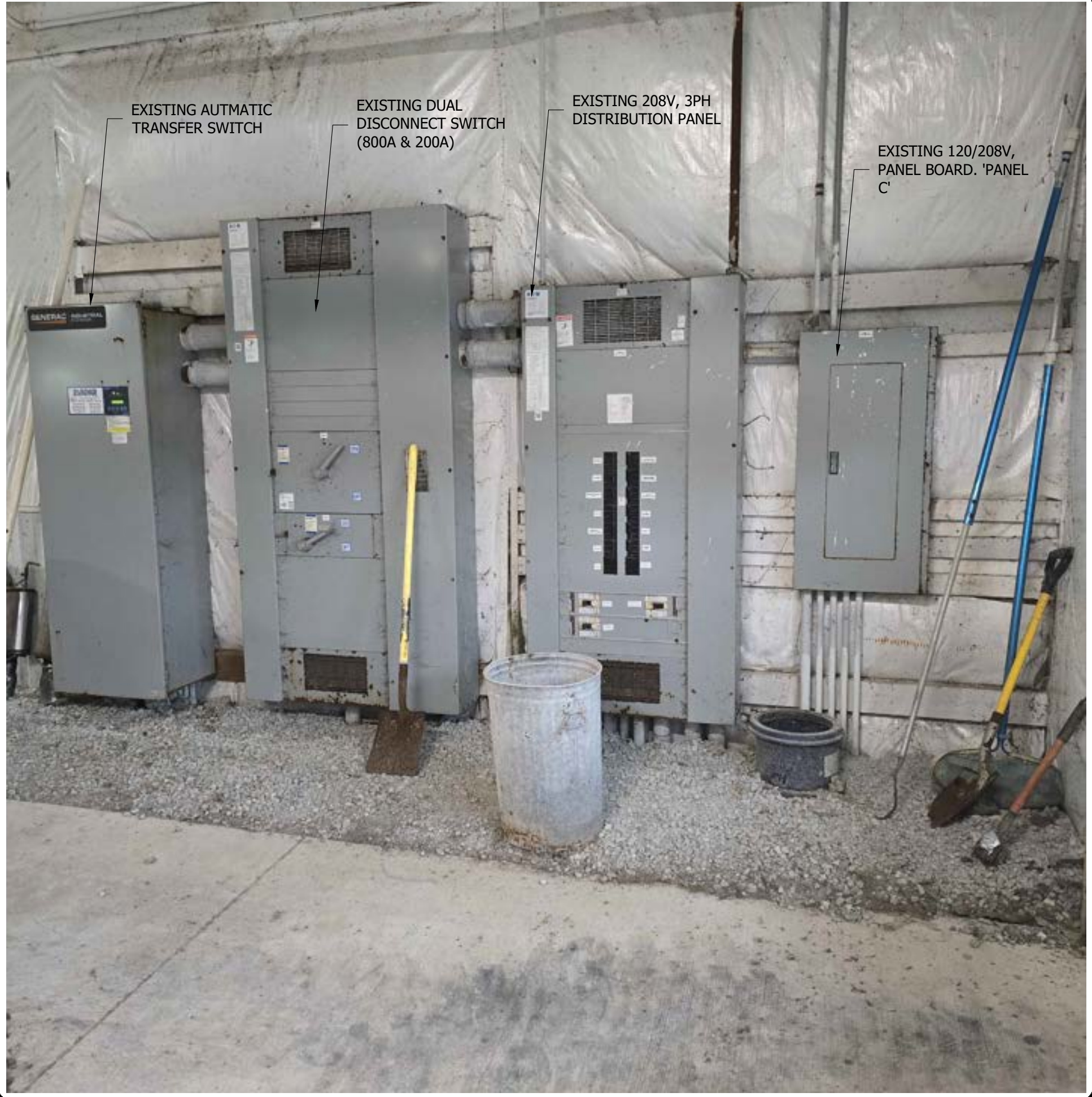
EXISTING POWER EQUIPMENT PHOTO - ALL TO BE REMOVED NOT TO SCALE
